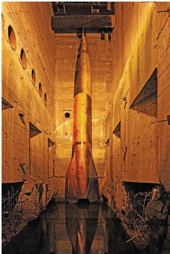
The life-size V2 shape shows where a door to a launch pad was planned. The reflection below is off water, the bottom 6m being flooded. Photo Bob Clary
